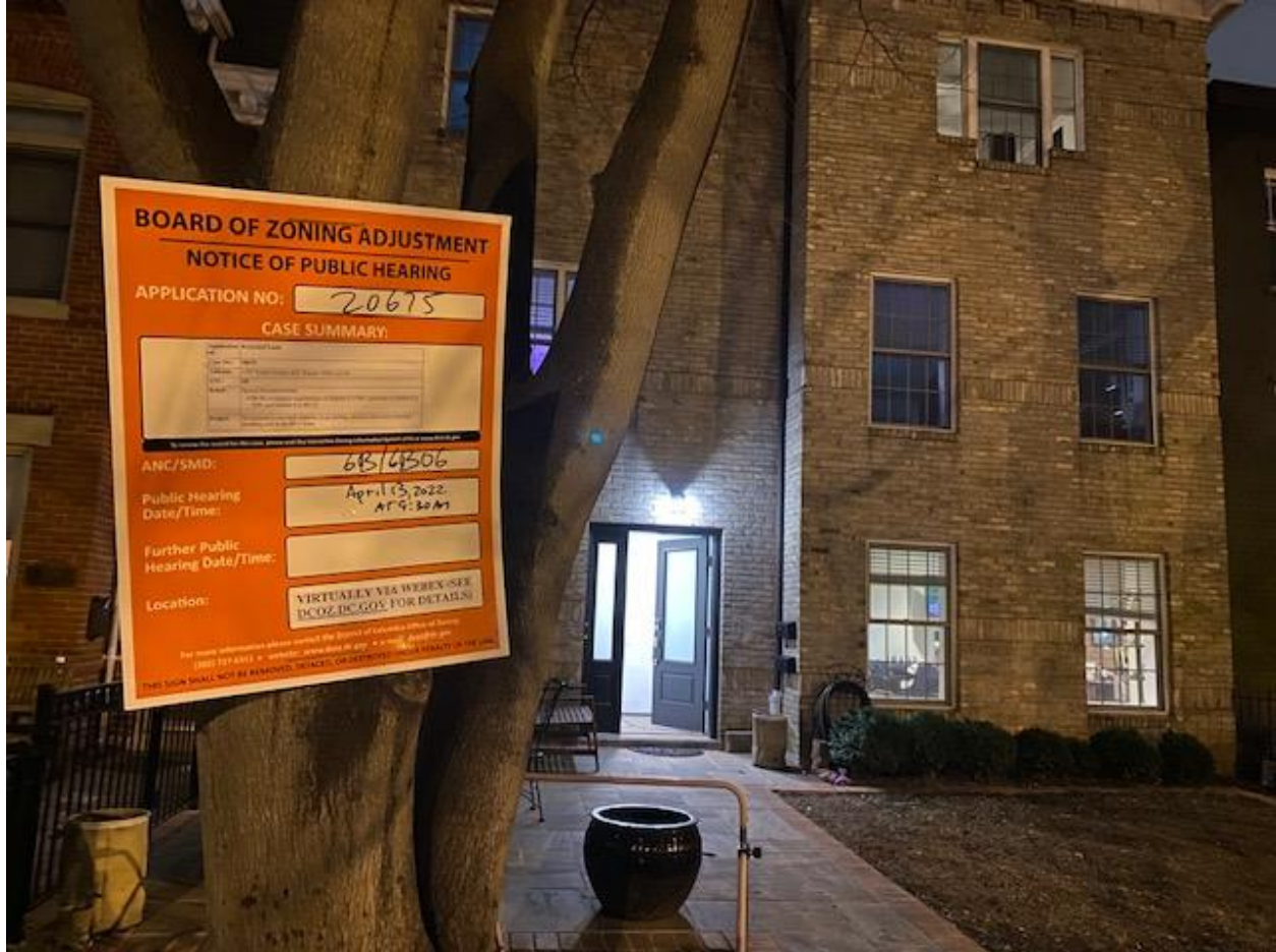
Photograph 2: From South Carolina Avenue, S.E.
